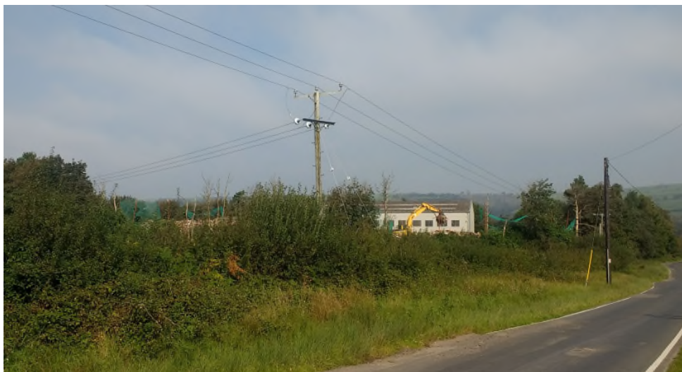
Fig. 5 – View of Site and Netting from Heol Llan
